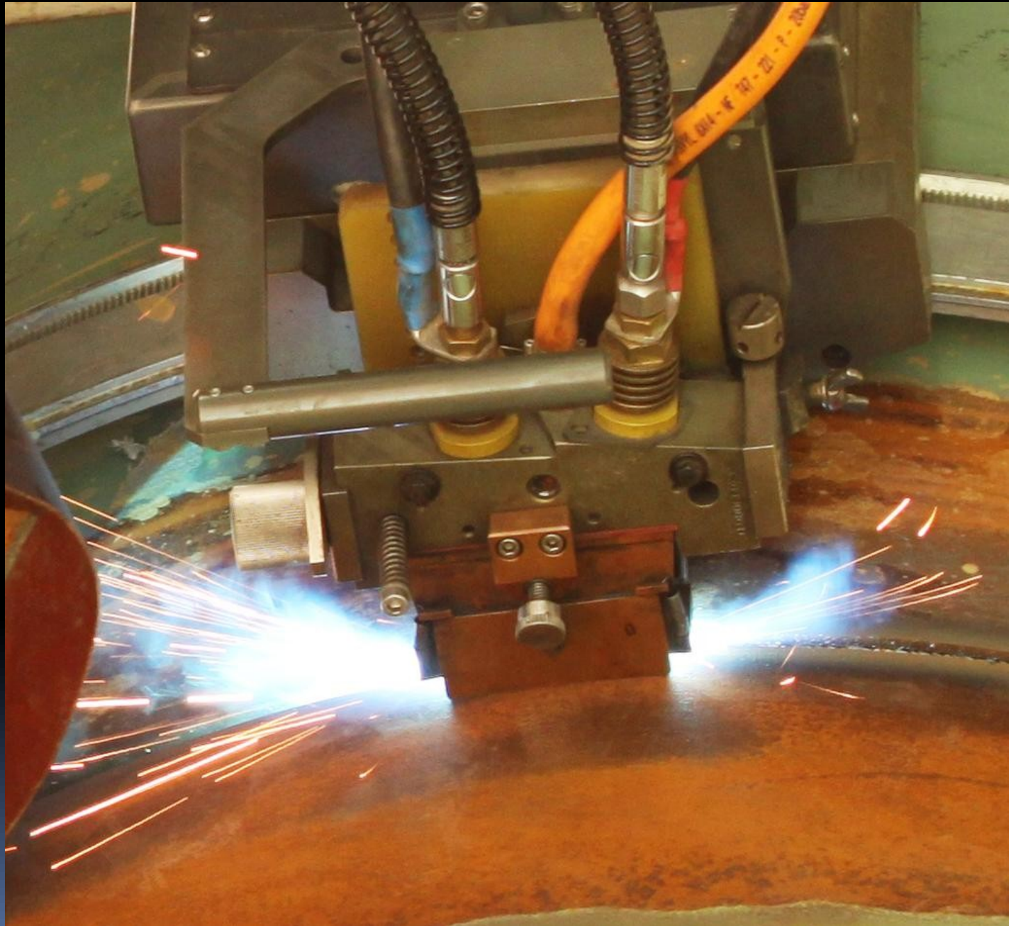
Automated Welding 42 Inch Pipeline
